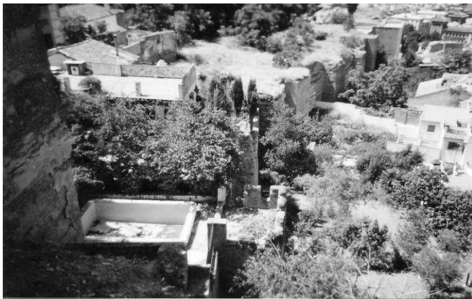
Figure 5. View from tower 8 to tower 14 before the restoration.
