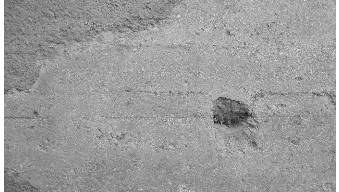
Figure 8. Detail of aguja and esparto grass trace on the tapia .
