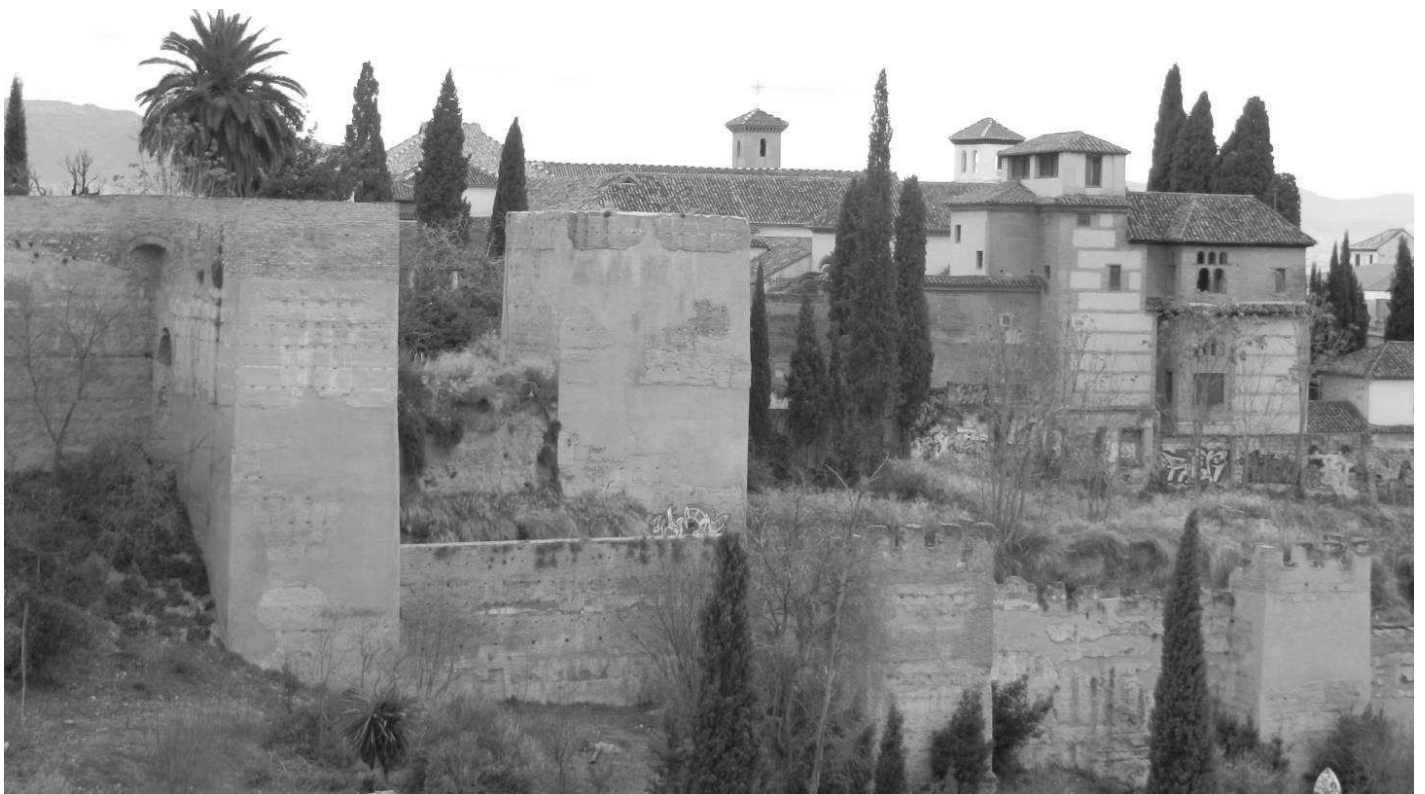
Figure 4. View of the central section after the restoration.
