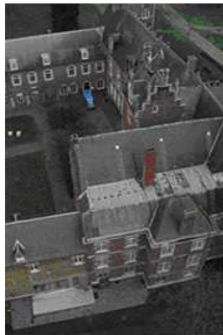
Figure 9: Complex roof structure of the Castle of Arenberg.
