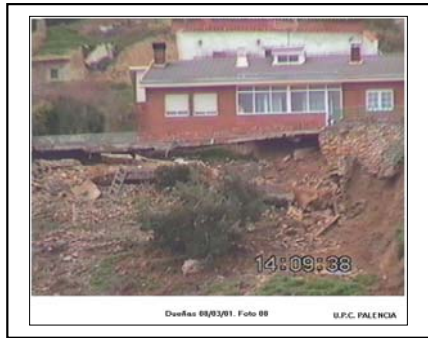
Figure.6. Landslide affecting a house foundation, during the March 2001 flood event (left). Figure.7. High water level affecting garages and basements in Valladolid (right).
