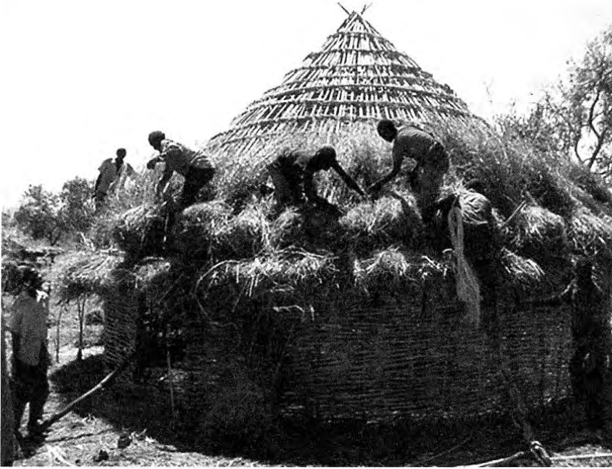
Fig. 6: Thatching a house through the amaha . Keshaf (Khomosha wereda ).
