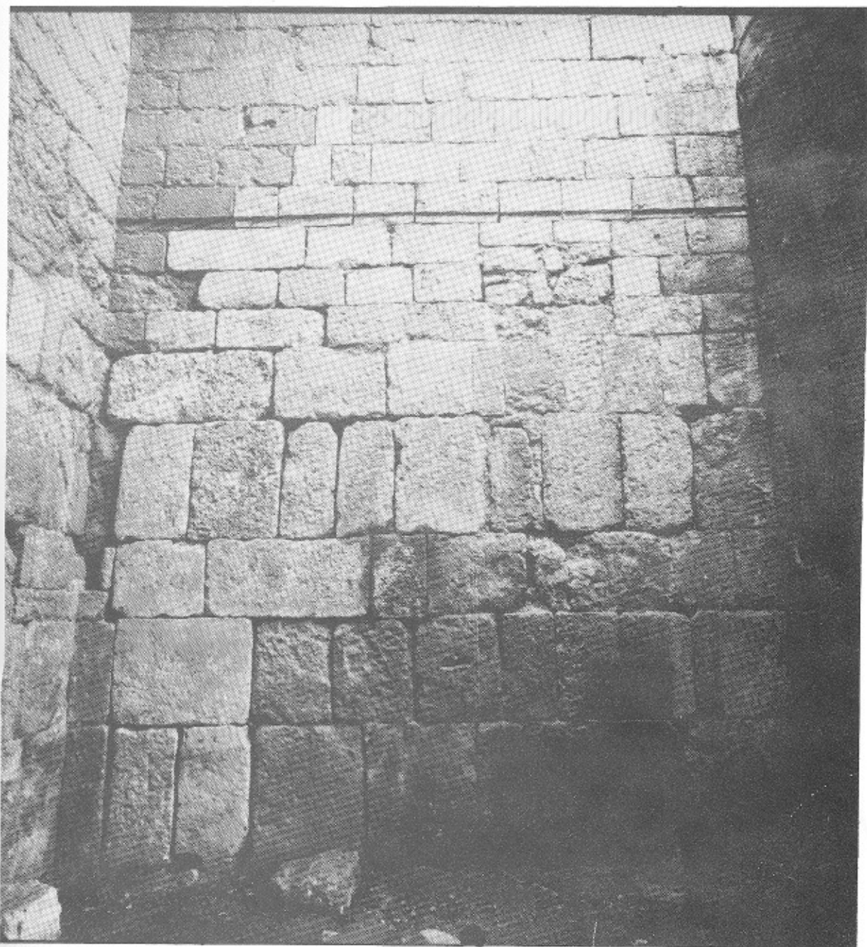
Fig. 4: The west wall of the northeast room after the restoration.
