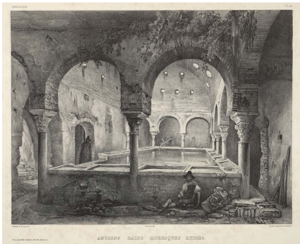
Figure 3: Warm room of El Bañuelo [1].
