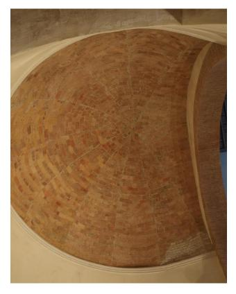
**Fig. 6:** Contemporary brick vault covering the counterapse of Mazote. Remains of the early medieval vault may be observed in the lower part of the image
