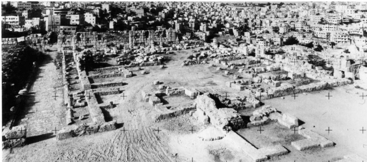
Fig. 27. Amman Citadel, Umayyad Palace. Building B after partial restoration.
