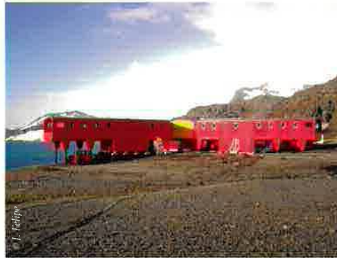
New accommodation module in the Spanish Antarctic Station Juan Carlos I.
