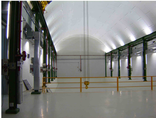
Figure 6.3: Main hall at Canfranc Underground Laboratory.
