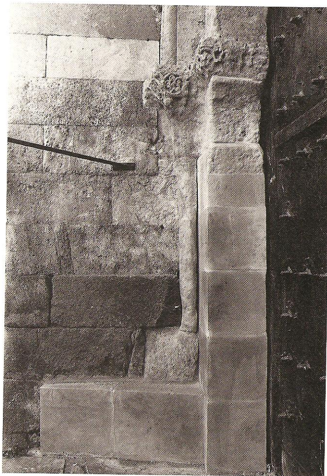
Plate 3.-Substituted ashlar.
