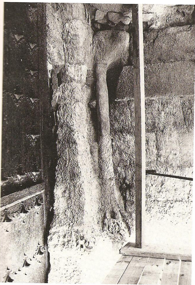
Plate 2.-Unworked ashlar of highly weathered jambs.
