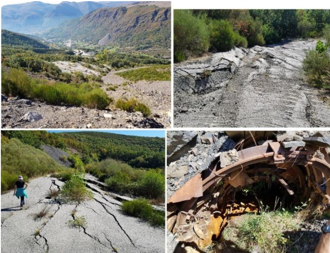
Figure. 2. Landslides in the Laciana Valley (León) induced by coal mining activity, a project led by OBTIER in agreement with the Junta de Castilla y León
