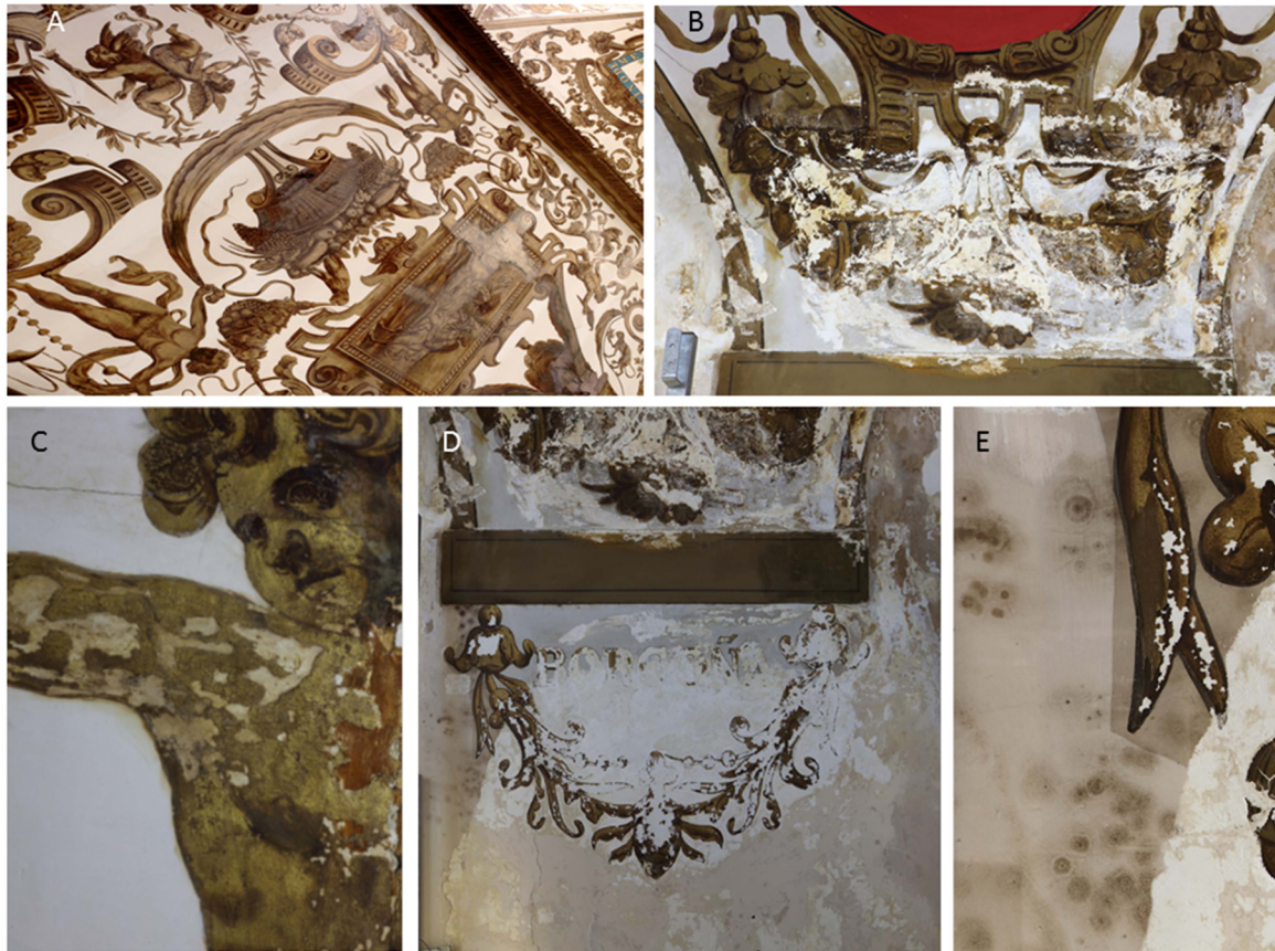
Figure 2. Salón de Reinos, Museo Nacional del Prado, Madrid, Spain. (A) Detail of the ceiling showing repaints. (B) Deterioration produced by a recent water leak. (C) Paint detachment in the ceiling. (D) Burgundy shield (sample M2) with fungal growth and painting detachments. (E) Detail of fungal growth in (D). Photos provided by Ágora S.L.
