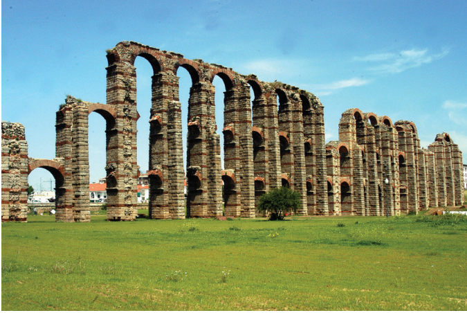
Fig. 4. Water conduit known as “Los Milagros.” By the author.
