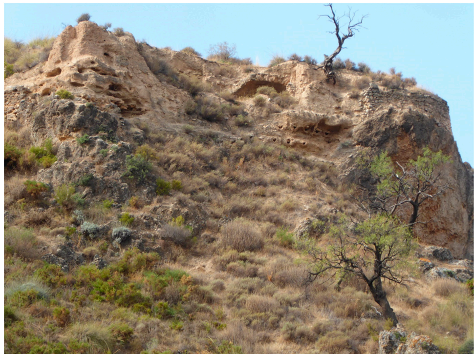
Figure 5. Exterior view of the north-western sector of the wall, Mondújar Castle. From this point, we can appreciate (on the left) the remains of the core of a rammed-earth tower and the ruins of the vault of the Andalusian cistern (in the middle), as well as the masonry plinth of the wall, to the right (A. Orihuela, 2020).
