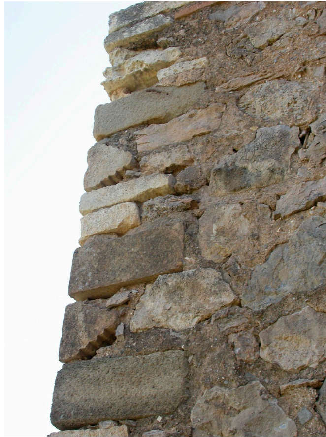
Figure 9. North-western corner of the tower gate, Mondújar Castle. In this picture, the stepped macabrilas can be appreciated (Antonio Orihuela, 2005).
