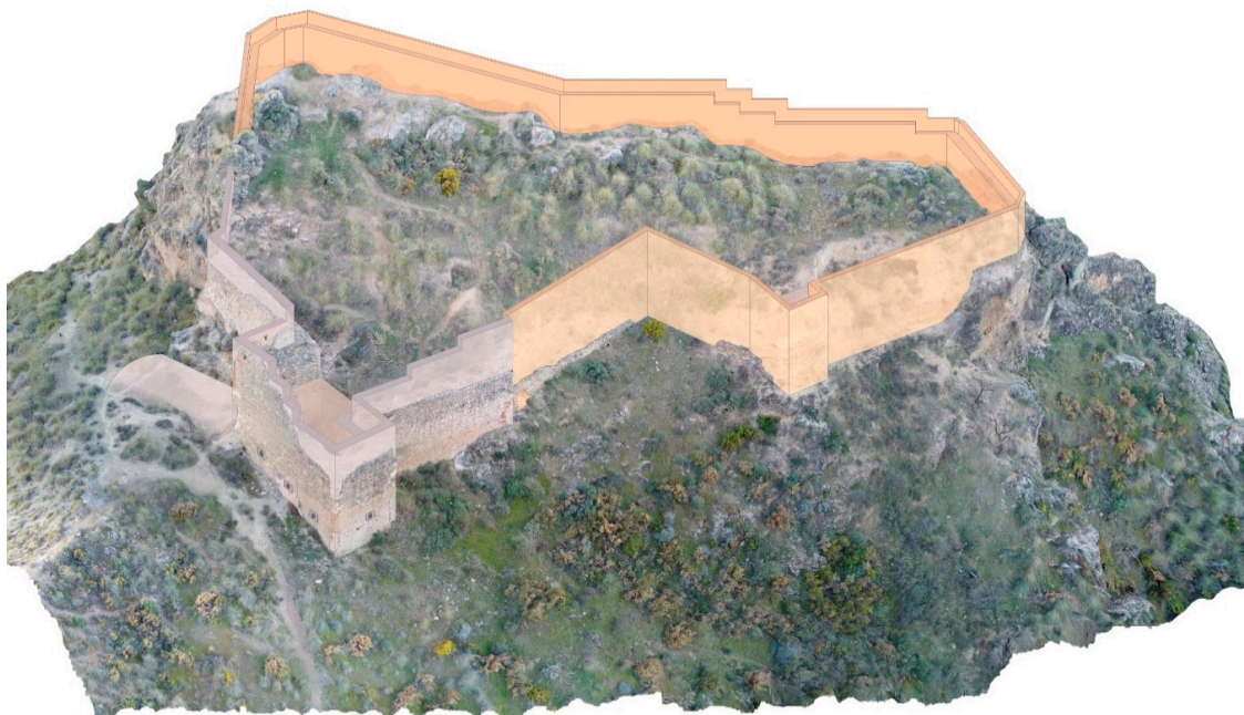
Figure 11. 3D digital mock-up of Mondújar Castle presenting our proposal of reconstruction of the ramparts (battlements not included). The Andalusí fortress has been drawn in ochre colour and the Castilian part in grey (Antonio Orihuela; Víctor Martín-Madrid, 2020).
