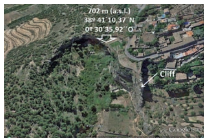
Fig. 1.- General view (Google Earth) of the collapsed dome of Barxell river waterfall.
